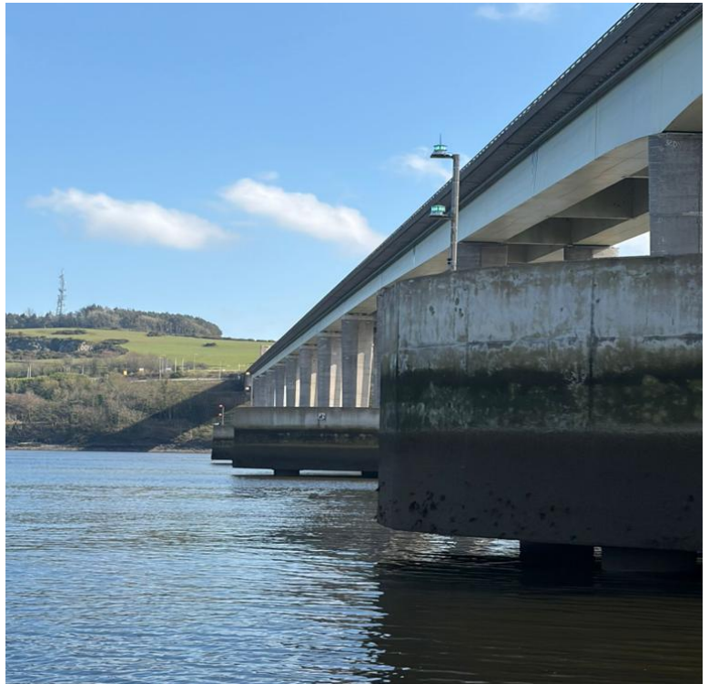
Bridge Pontoons showing green, yellow and red marker lights at navigation channel
